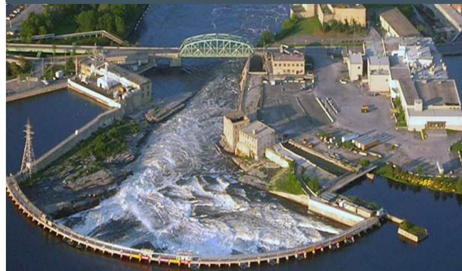
Chaudière Vertical Flip, Ontario, Canada
