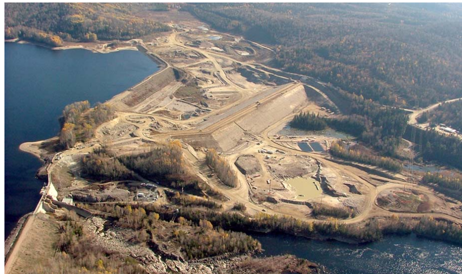
Shikwamkwa Replacement Dam, Ontario, Canada
