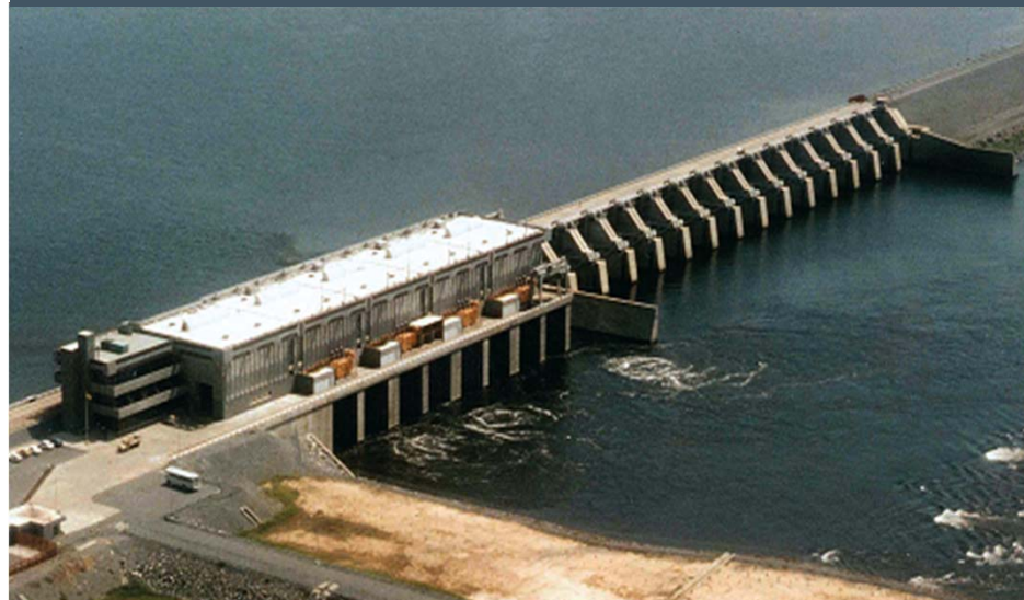
Kpong GS Rehabilitation Project, Ghana
